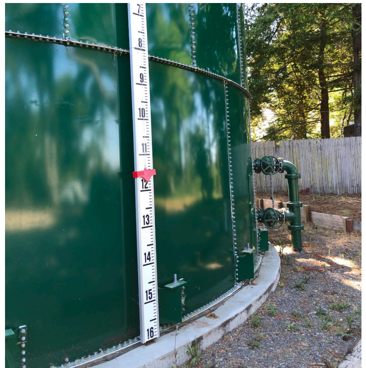
This 55,000-gallon water tank in Seahaven is one of nine tanks comprising the Inverness Water System. The gauge on the 16-foot tall tank shows it is about three-quarters full. Water in the tank flows out through the big pipe on the right into the main on Via de la Vista. Normally, only the top valve is open, which is about one-quarter of the way up from the bottom of the tank, so even if the tank empties all the way down to that valve's level, 25% of the tank's capacity is held in reserve for fire and other emergencies.
